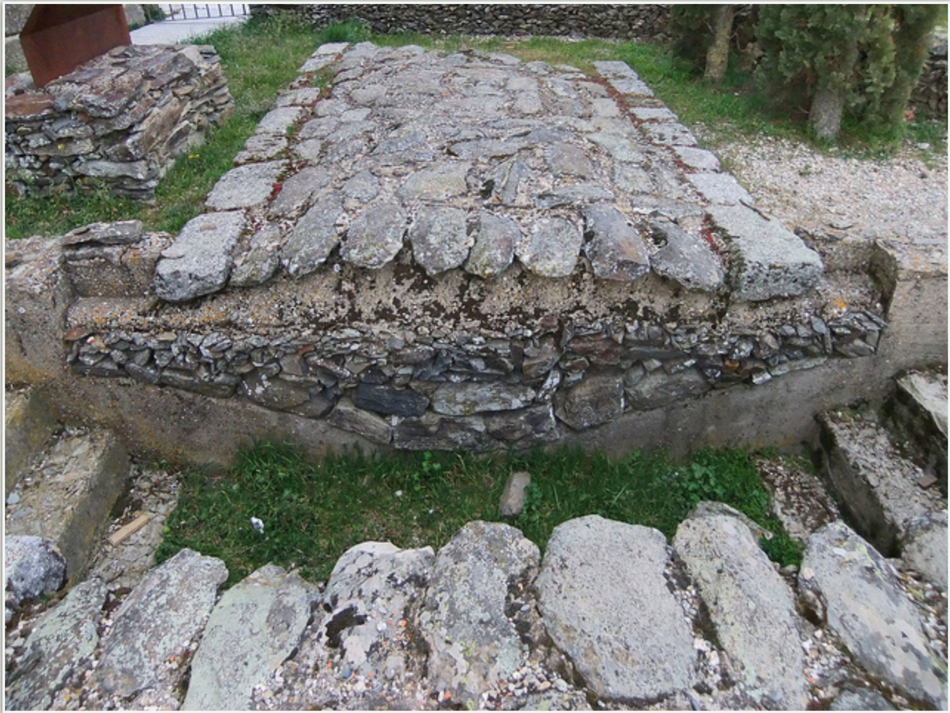
Cross-section of a Roman road in Fuenterroble, Spain.
